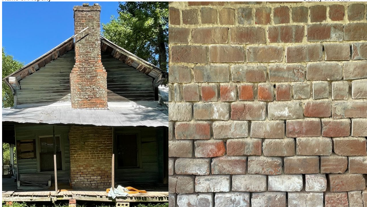
Figure 08. Chimney and close up of brick courses at Benson house.
