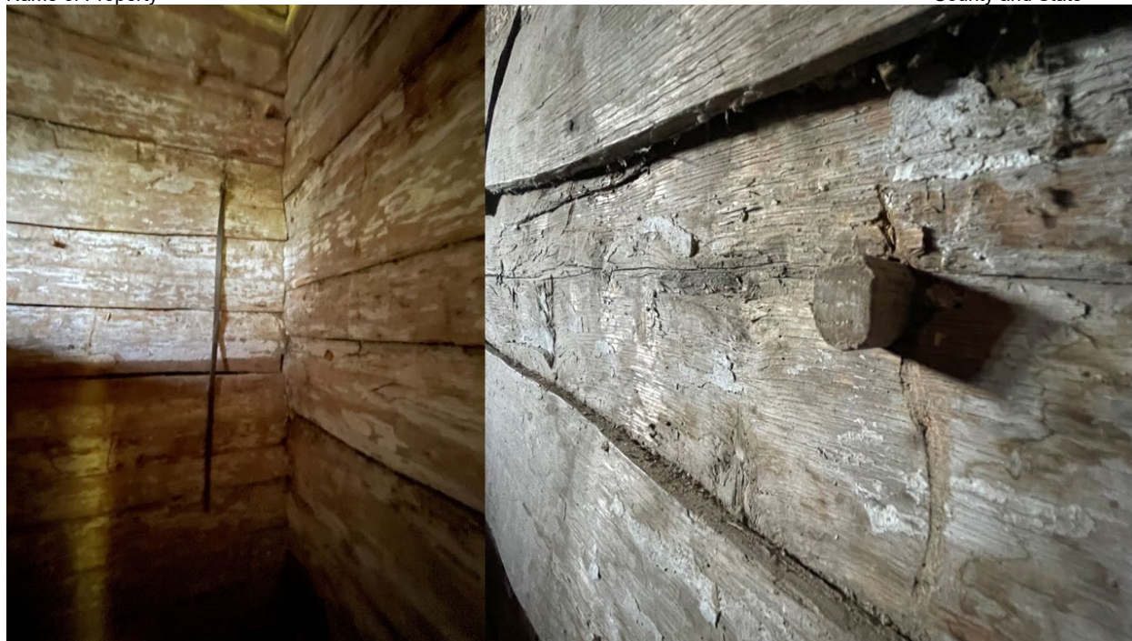
Figure 06. Plank log construction (left) Peg protruding from log (right)
